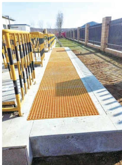
Nullah alteration of Avanc Pharma
